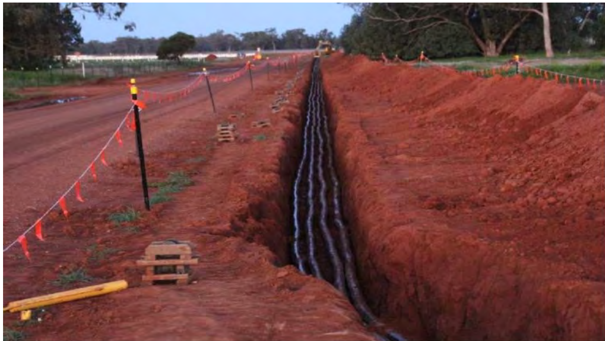
Figure 3: Typical cable trench for MV collection system
